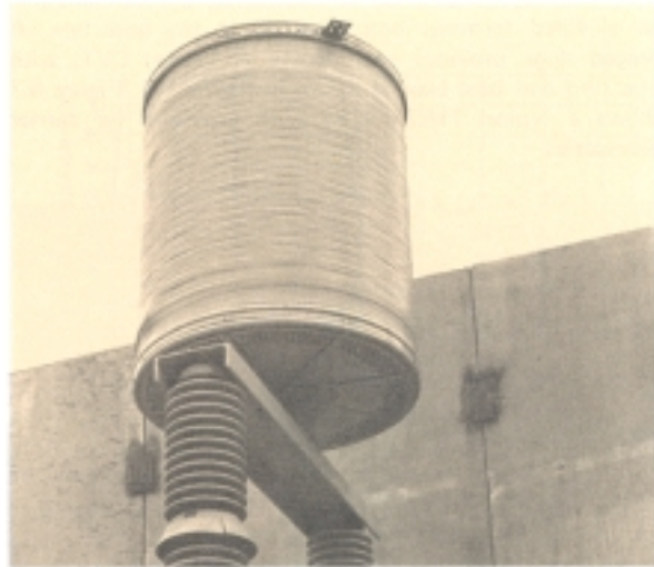
Figure 6.5. Line trap, rated at 2000 amperes, 0.35 mH, 230 kV, using a horizontal-channel mounting. This keeps the axis vertical for optimum cooling.
