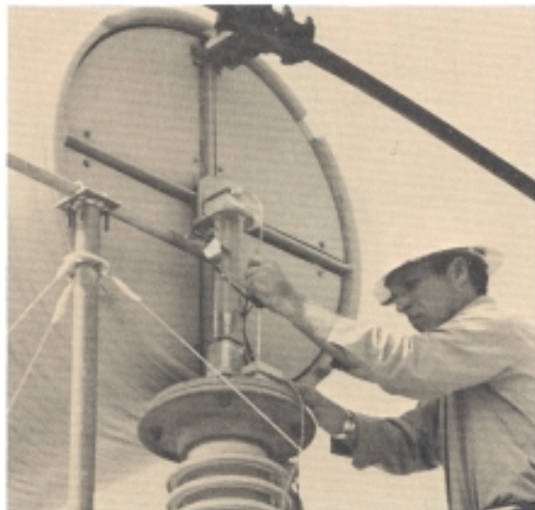
Figure 6.6. An 800-ampere, 0.265-mH line trap being installed in the horizontal position.
