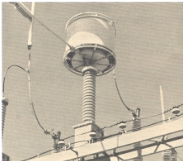
Figure 6.4. Line trap mounted on capacitor voltage transformer.
