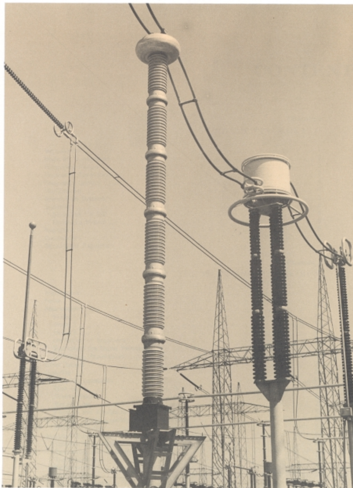
Figure 6.9. 735-kV capacitor voltage transformer and 2500-ampere, 0.7-mH line trap, as installed at Hydro Quebec's Duvernay substation.
